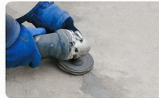
1 Surface Preparation Clean + repair cracks
